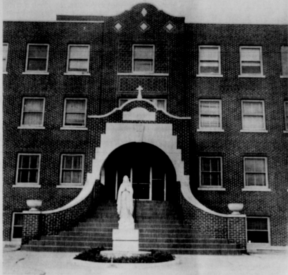
MERCY HOSPITAL — Slaton Rotary's number one service project.
