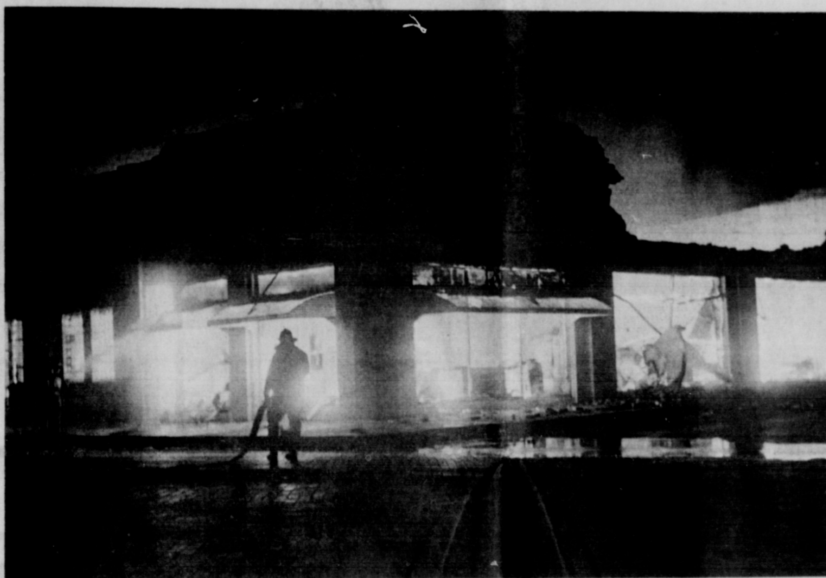
FIRE IN THE NIGHT — This building at the corner of 9th and Lynn Sts. in downtown Slaton burned in the early morning hours Saturday, with the blaze too far gone to be halted when it was discovered about 2 a.m. Firemen were on the scene all night. The building housed Western Hog & Cattle Co. and Hailey's Auto Repair, both of which were total losses. The estimated $160,000 loss made it the costliest fire in years in Slaton. (SLATONITE PHOTO by Dalton Wood)
