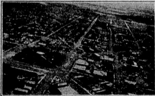
A PARTIAL VIEW OF SLATON FROM THE AIR Showing the City Hall in the center of the block, with one of the finest lawns in West Texas. Shade trees and shrubbery form a background for the building.
