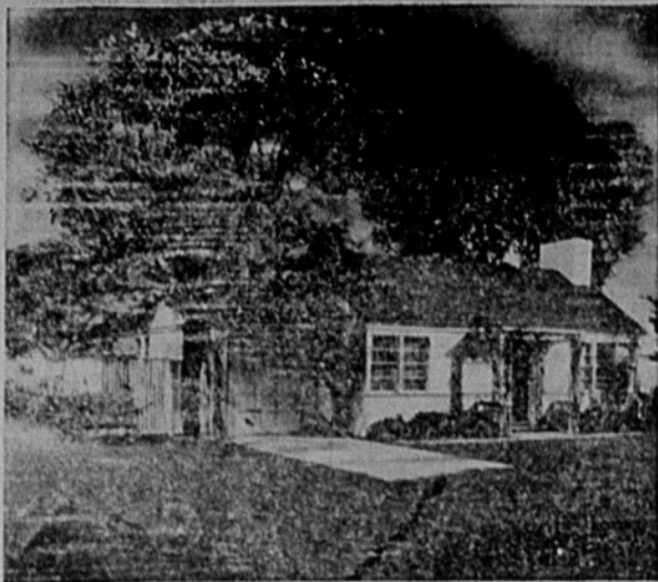
A cool court is one of the many pleasing features of the modern low cost home shown above as pictured in the July issue of Good Housekeeping magazine. Bright, breeze-swept rooms, pleasant views through spacious windows and a step-saving plan are other features that make this house a happy solution to the housing problems of many average American families.
