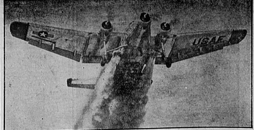
NEWEST LIGHT TRANSPORT —Six jet rocket units and three engines enable the U. S. Air Force's newest light assault transport to take off in a space of less than 500 feet. Weighing 20 tons, the Northrop Raider C-125 was designed to transport heavy loads in and out of small, unimproved clearings. The photograph was made during one of the ship's test flights at Hawthorne, Calif.
