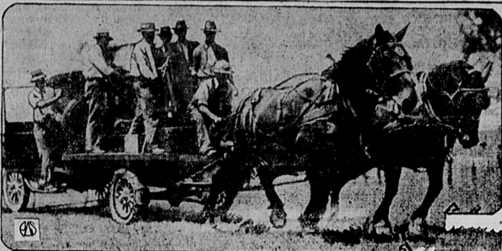
"Bill" and "Colonel," the 3,800-pound team belonging to George Wilcox, of Greenville, Ohio, pulling against a motor truck, at the Jay County, Indiana, fair, made a record of 3,550 pound drawbar pull, equal to hauling 46,102 pounds on a wagon of eight fourteen-inch bottoms cutting a furrow six inches deep.
