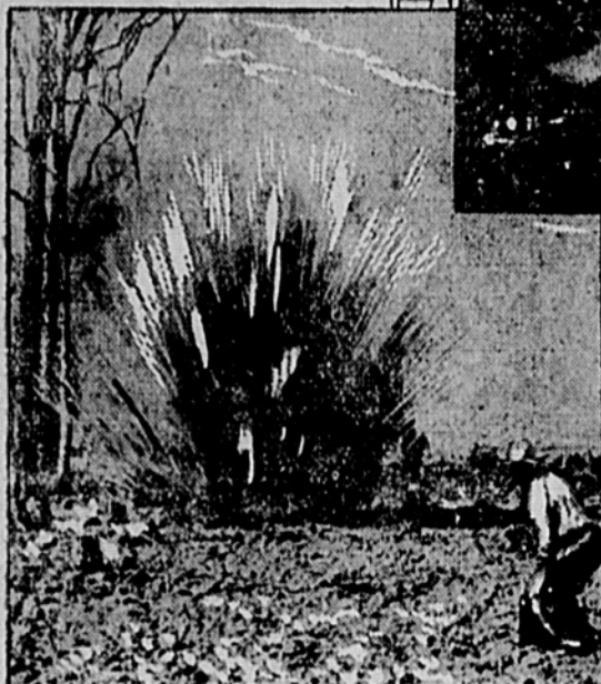
Firing a dynamite shot with an electric blasting machine.
