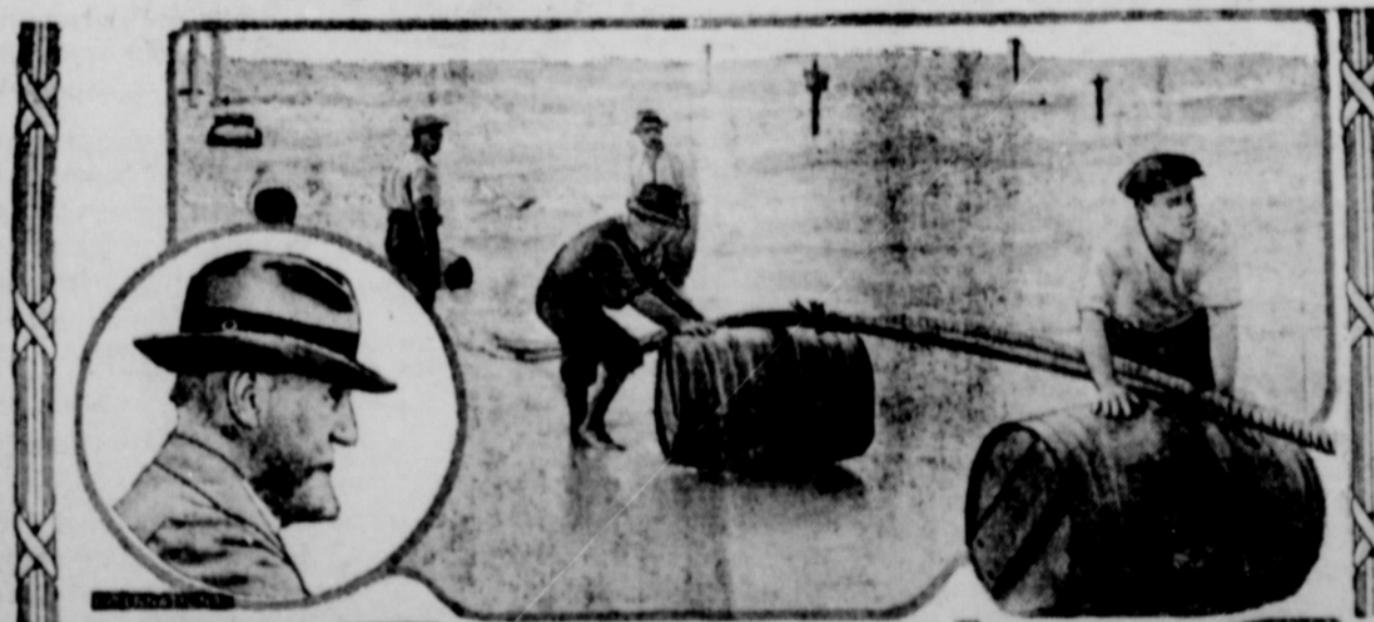
The American shore end of an entirely new type of submarine cable, which will transmit signals at several times the speed of any long cable now in existence and which will utilize important new discoveries in electrical science, was landed at Rockaway beach, New York, the other day. The illustration shows the workers bringing in the cable end, and, at the left, watching the operation, Edward Morse Field, whose father laid the first transatlantic cable.
