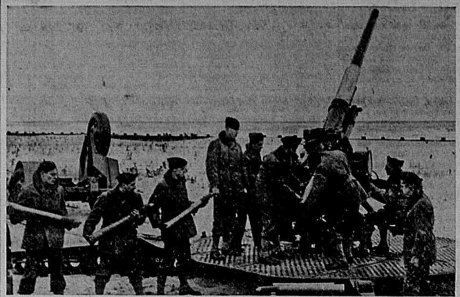
National Guardsmen of Battery D, 212th coast artillery unit, only National Guard anti-aircraft unit in New York state, load a three-inch, super-powered gun, one of 325 ordered by the government. The new weapons, which would defend New York city in case of air attack, have a three-inch bore, fire a 28-pound projectile containing 253 one-half-inch lead pellets, and can fire 30 shells a minute. Guns were tested at Fort Tilden, Rockaway beach, New York city. It was the first time since 1917 that a N. Y. National Guard regiment held winter maneuvers.
