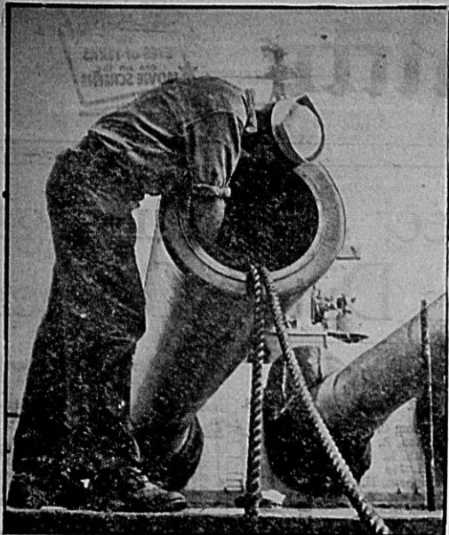
BORE CHORE —Following a prolonged shelling of Communist installations and supply centers, a crew member of the USS New Jersey makes himself busy in this Navy photo cleaning the bore of one of the super-dreadnaught's 16-inch main battery rifles. The "Big Jay" has played an important, deadly part in land-bombardment actions off Korea's east coast.
