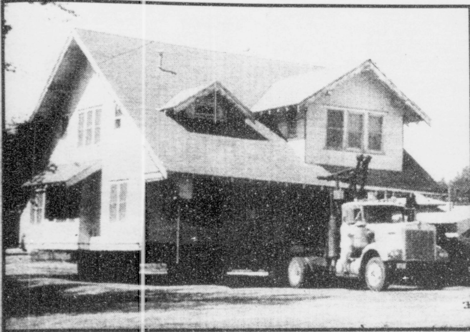
While Kathleen and Keith and crew mover their new home into town, eager onlookers anticipated the new arrival of the newest addition to the neighborhood. While the new home comes into town, X-cal Electric Company raise the highline wires so the new home can make it's way down Old Rt. 66 to finally settle on it's final resting spot. McDowell Brothers House Movers Inc. with keen professionalism, moved the house with ease. Picture & caption by Caty Wilson Koetting
