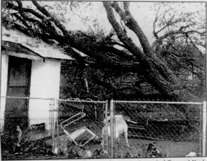
Weekend storms with strong winds uprooted a tree in the yard of Trey and Vonda West causing some damage to the roof.
