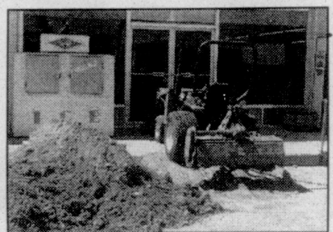
Work on The Groom Grocery Store continues.
