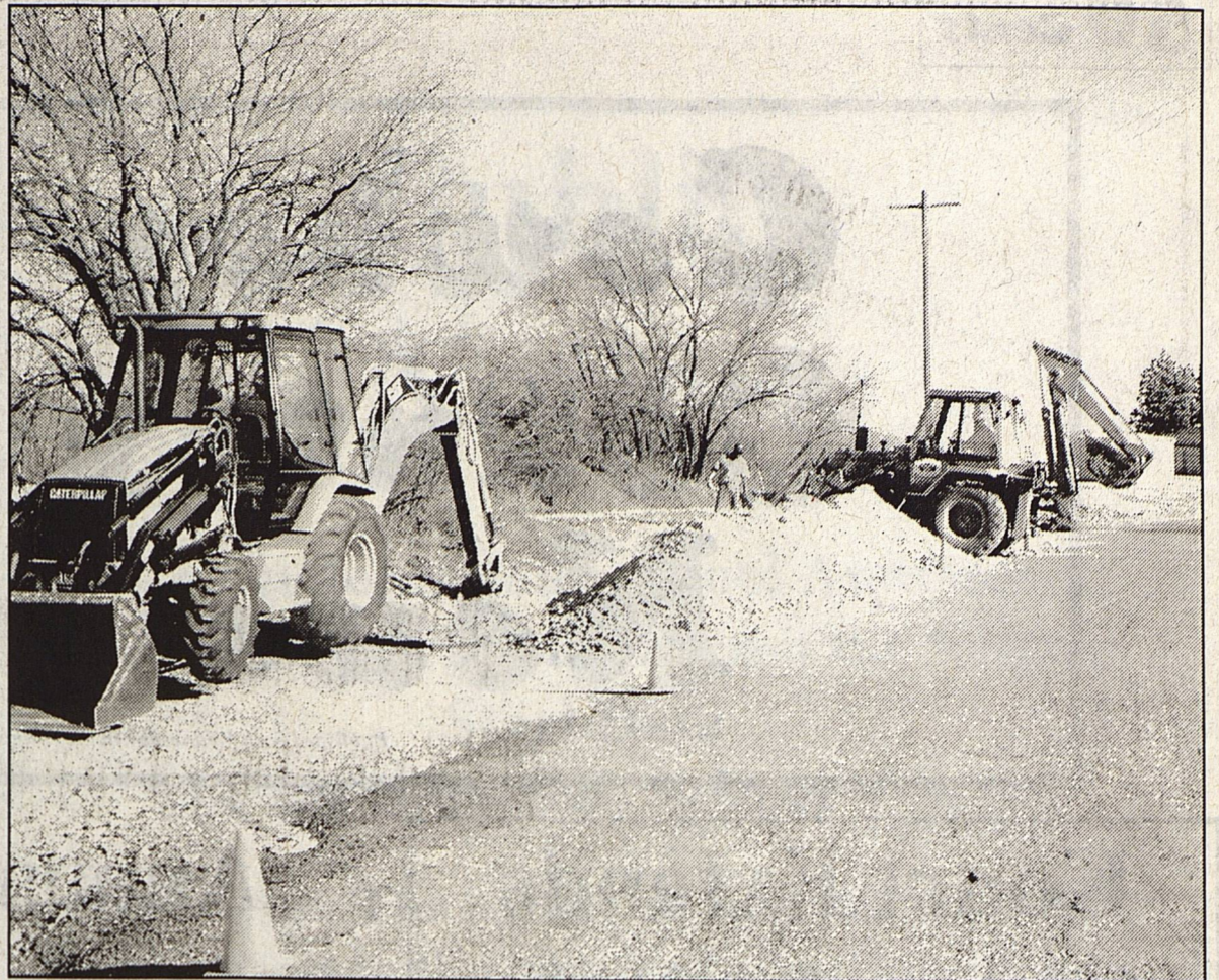
City employees Alex Barrientes, Jerry Dominguez and Ryan Martinez worked last week replacing a septic tank on the north end of Copeland Avenue with a new sewer line. The work is continuing the City's project of replacing all old septic tanks. This new line will extend to behind Sacred Heart Catholic Church and then down hill to the city lift station. The pumps there were under water in the Fall of 2004 during the brief flood, and will be raised some eight feet when the new line is tied in.
