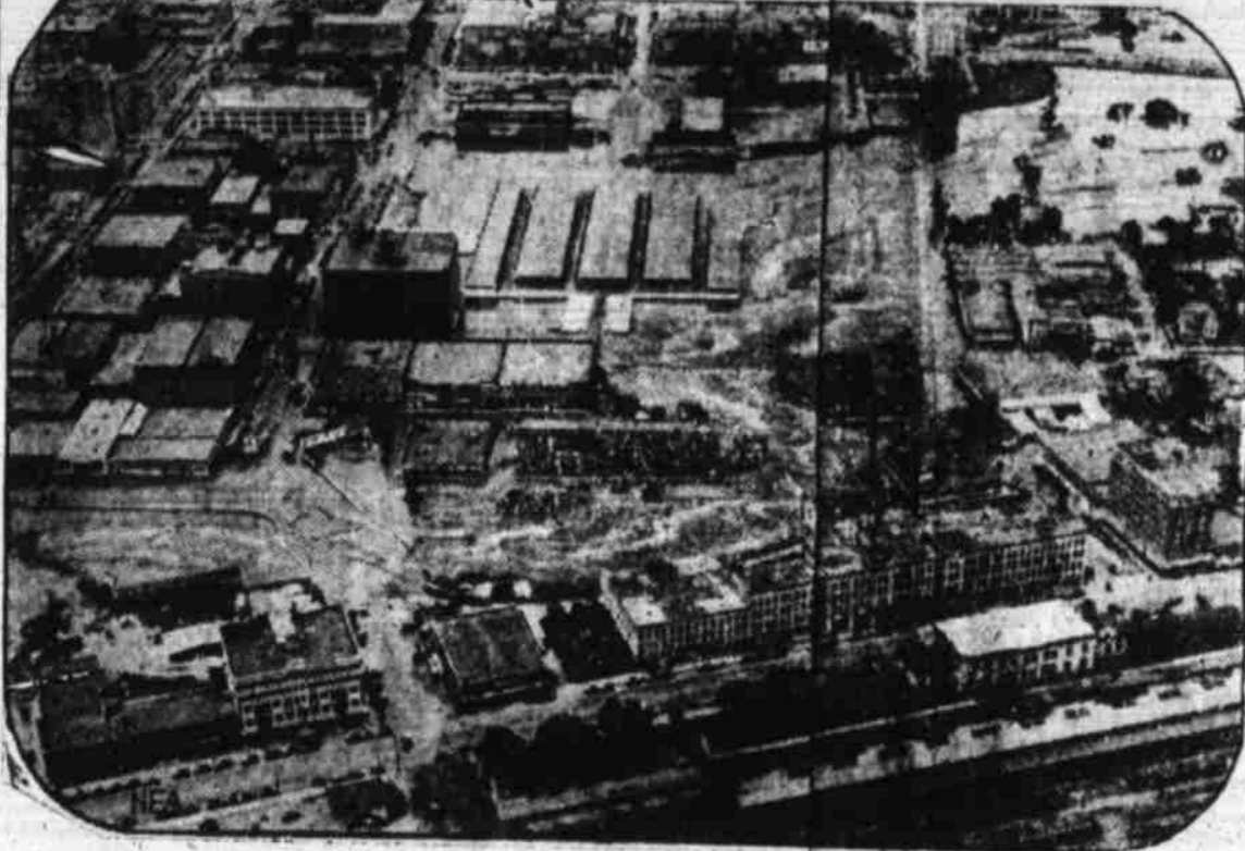
A remarkable airplane view of the flooded district of Houston, Texas, is shown above. Water from Buffalo Bayou, which became a rushing torrent when swelled by recent rains, rose nine feet in six hours and caused thousands of dollars of damages. The city asked for typhoid serum, the drinking water supply being cut off.
