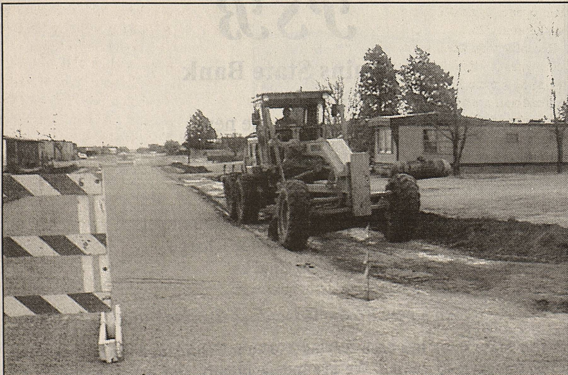
County motor grader removes dirt for street resurfacing
