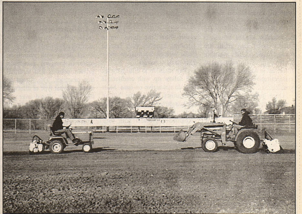
PISD employees Robert Loya and Shane McKinzie shown tilling in clay on infield
