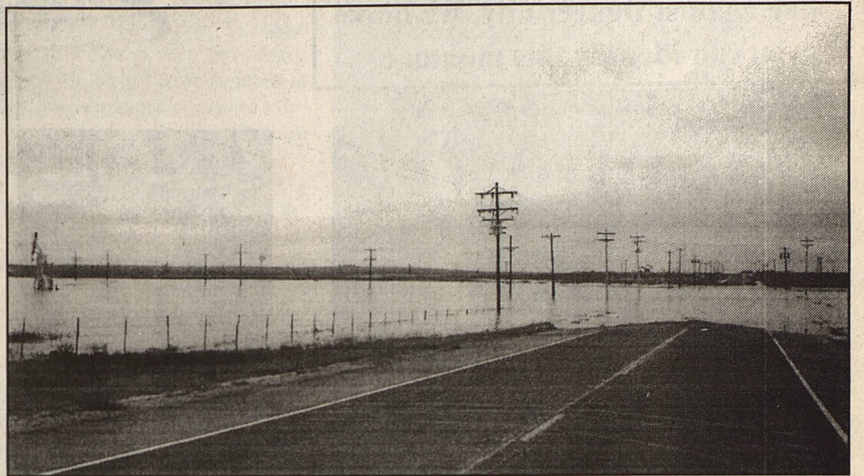
US 380 to Roswell closed until Thursday, under water many places between here and Bronco
