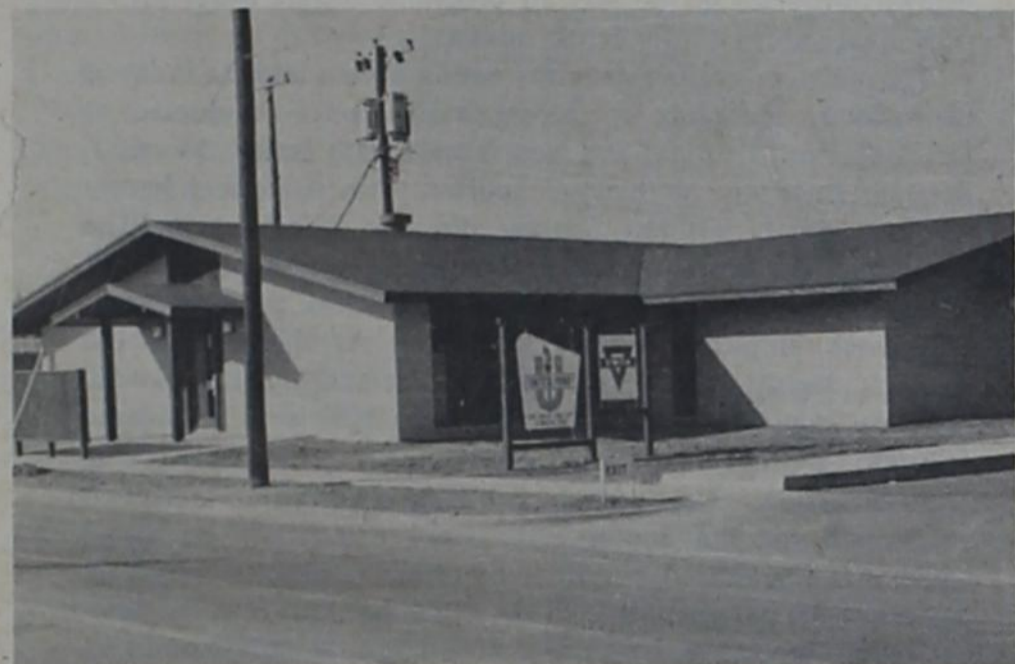
Dedication services are scheduled tomorrow evening for the new YWCA building. Ceremonies are scheduled for 7:30 p.m. Friday for the formal dedication of the new $80,000 headquarters at 3101 35th Street for the Young Women's Christian Association of Lubbock.
