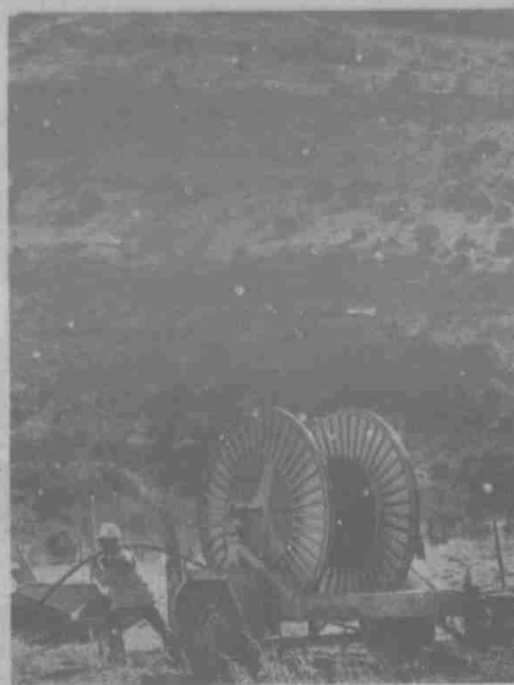
Southwestern Bell will lay several hundred miles of underground cable in
