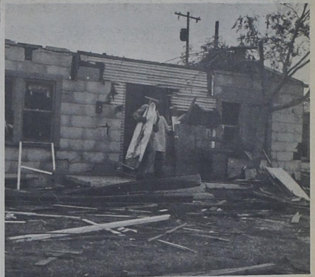
More Storm Damage—Tuesday morning clean-up was in full swing for this couple as they helped remove valuables from a house on 6th St.
