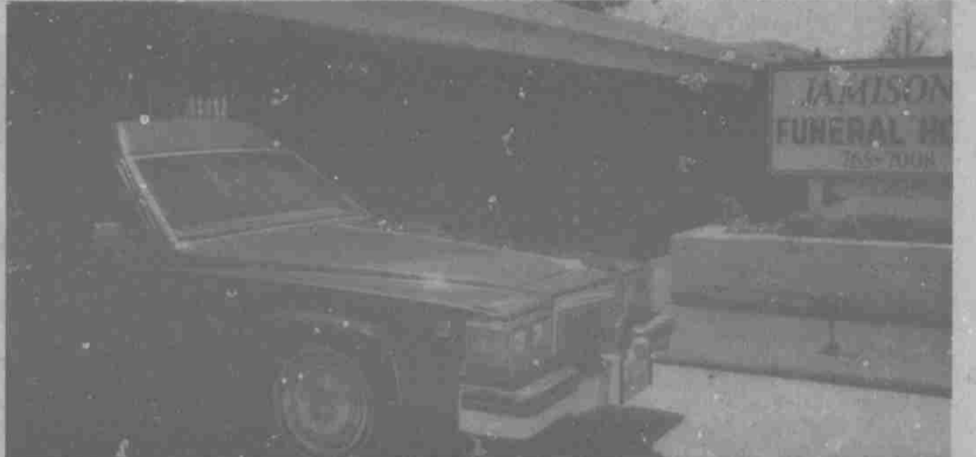
Picture 5 - The present facility in Lubbock, built in 1971
