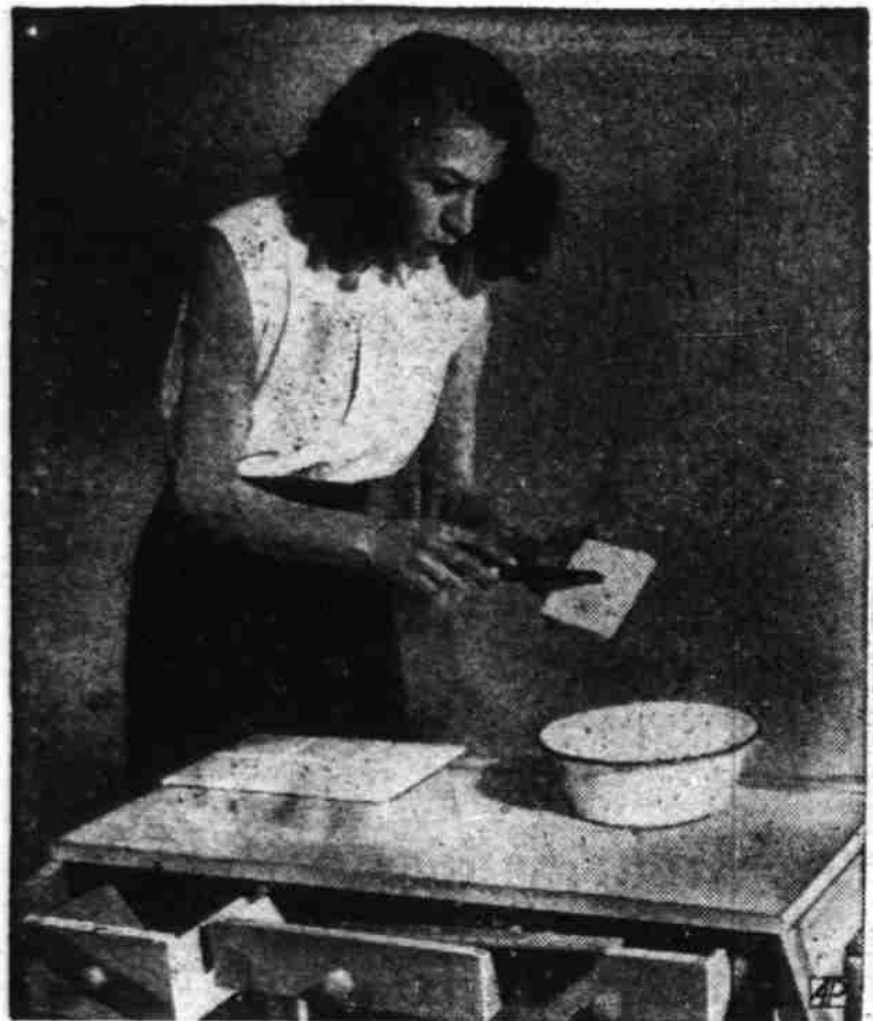
TILE FOR TABLE TOP —Trying out an idea of her own for a dressing table top, Ann Edman of New York "butters" a square of glazed tile with bonding compound preparatory to cementing it to the wood.
