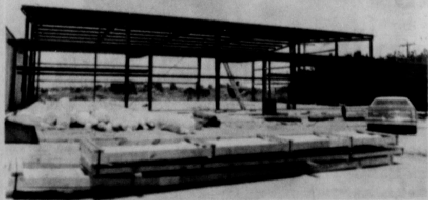
PROGRESS AT Wood-Jordan
