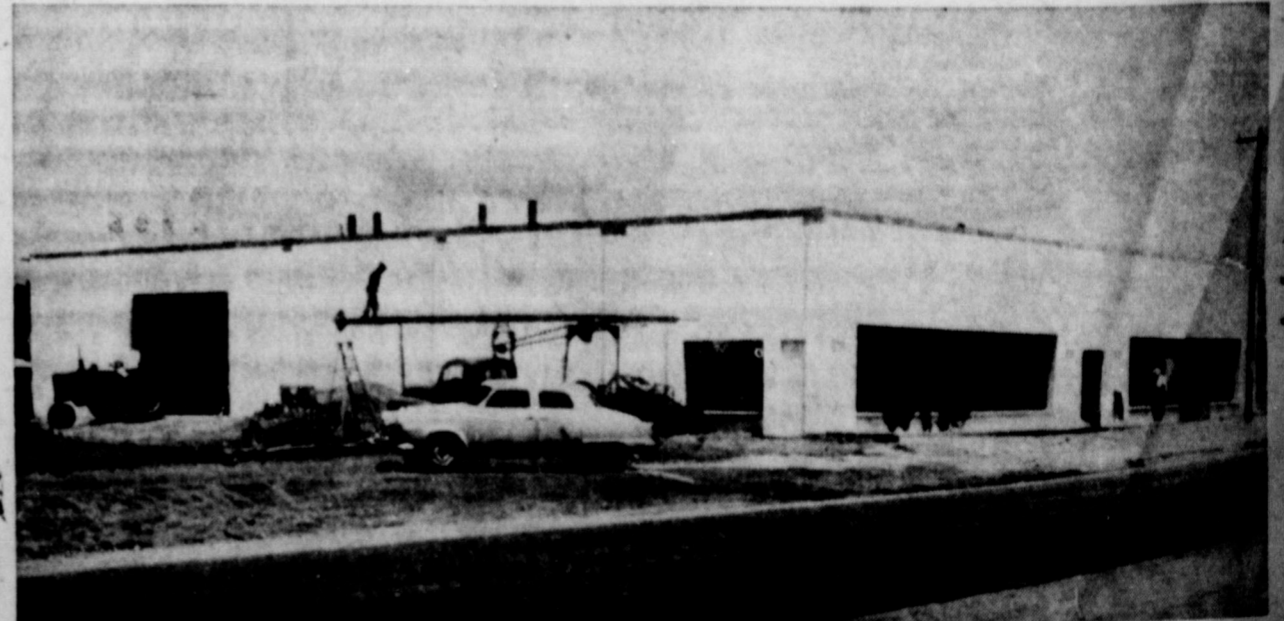
WORKERS WERE BUSY completing Earth's largest business building when the above picture was taken this week. The new 100' x 100' structure owned by H. L. Dent, will be the new home of Dent Implement and Hardware Company, Earth's John Deere Implement dealer.
