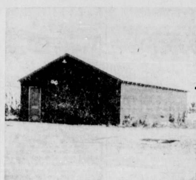
THE NEW Oddfellow building recently constructed in Earth is located on the west side of Main street. Although the exterior of the building has not been completed, it is now being used as a meeting place for the lodge. (Photo by Taylor Studio, Littlefield)
