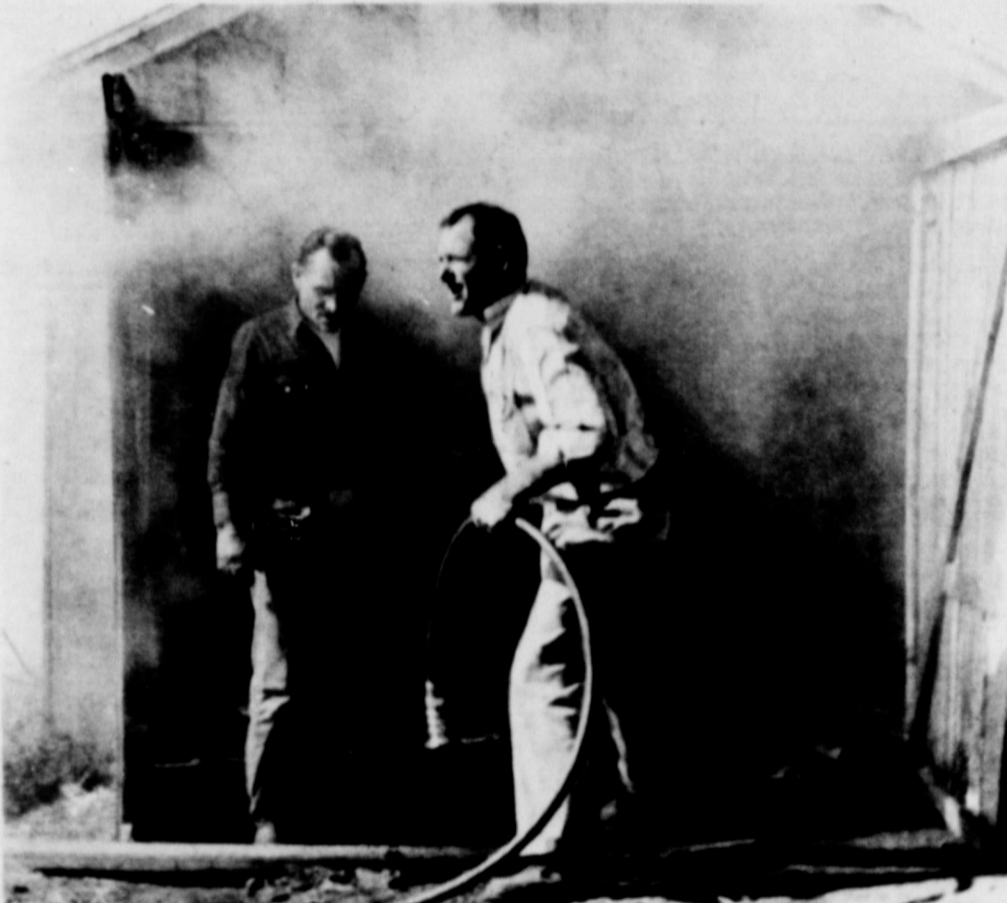
GARAGE SUSTAINS MINOR DAMAGE... Volunteer firemen were credited with prevented heavy damage in a fire Monday, shortly after noon, which threatened to destroy the frame garage owned by Jack Hadaway and located south of the Texaco station. Trash blown from a burning trash barrel north of the garage is believed to have started the blaze. A divan on the south side of the garage was completely destroyed. Shown here are Fire Chief Donald Layman and volunteer fireman Harold Britton.
