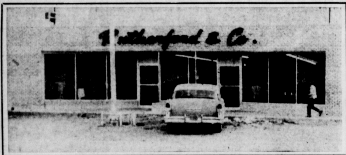
Our new building was completed in late September. We began our move from Littlefield to Earth immediately. The formal opening was held Saturday, October 22, 1955.
