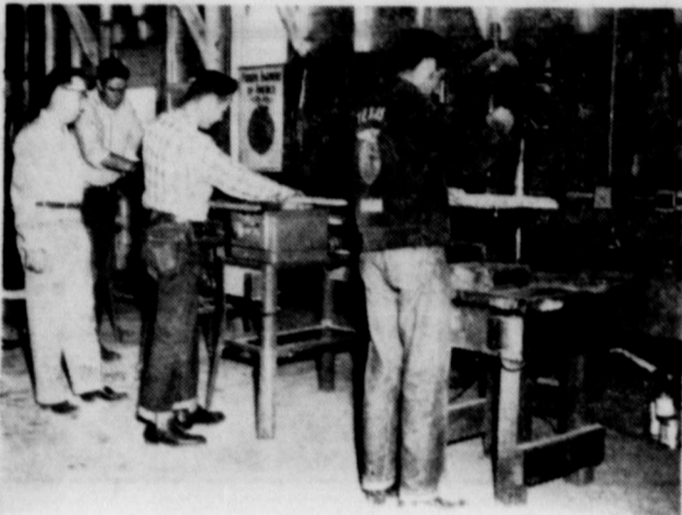
John Dwyer, Vocational Agriculture Instructor, Groom, Texas, observes as students of Vocational Agriculture operate properly protected electric power tools. The wiring system is planned and adequate to supply the motors with sufficient electricity. All of the equipment has grounding protection. From the left: John Dwyer, James Angel, Ronald Homer, and Donald Mansel.
