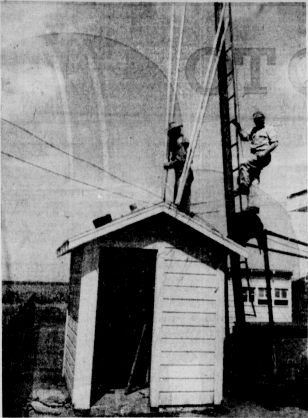
HERE ARE Clyde Parish and Fuzzy Martin setting a pump at the Troy Blackburn farm, 6 miles north and 1 three-fourths east of Springlake. This pump setting is another of the many services by the Dent Farm Supply that will have their formal opening today and tomorrow.
