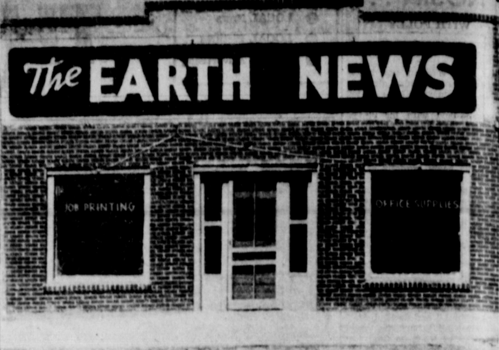
PARTITIONS were moved and painting completed this week in this building on West Main which will house the offices and shop of the Earth News. The News office will be moved from its present location into the new building as soon as a telephone is installed. Printing equipment is due to arrive within the next week or two. (Staff Photo)
