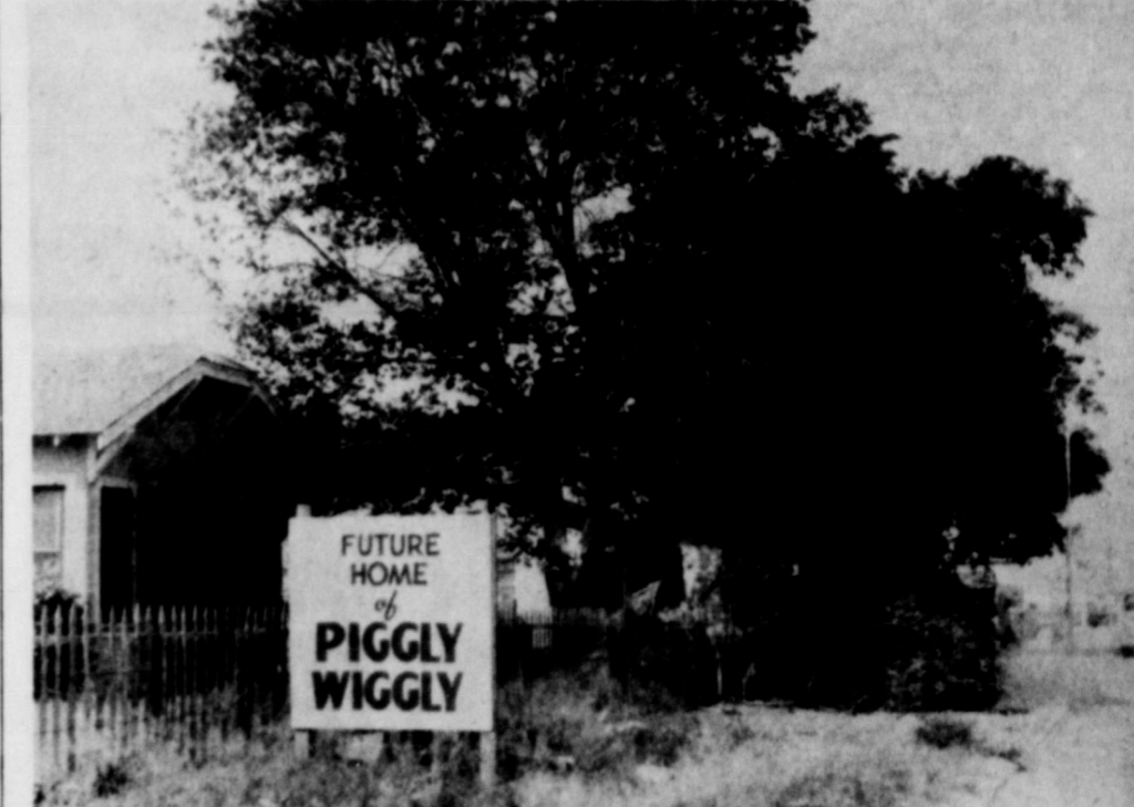
FUTURE HOME OF PIGGLY WIGGLY---This sign designates the site of the modern new supermarket to be constructed in the near future. The two houses shown here are being moved today to new locations on 4th Street. Dutch Been, who will be owner of the new building, will sub-lease to the Piggly-Wiggly Chain.
