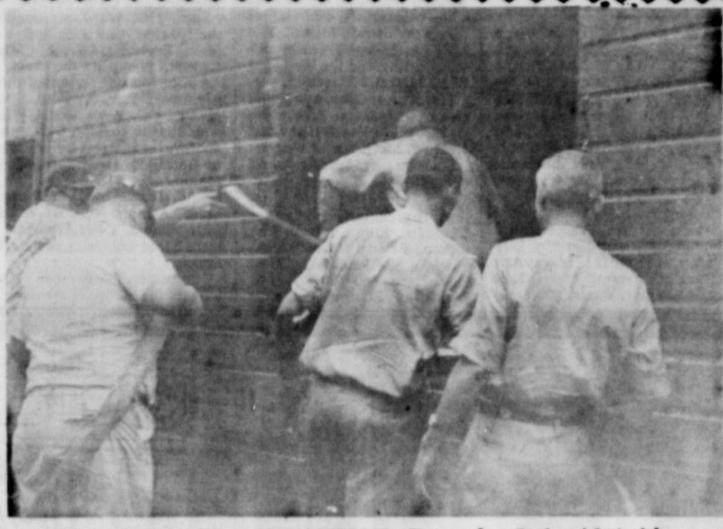
CAIN HOME DAMAGED BY FIRE SATURDAY ---Firemen from Earth and Springlake, hampered by dense smoke, succeeded in saving the farm home from total destruction. Firemen are shown entering the bedroom, where the fire is believed to have started.
