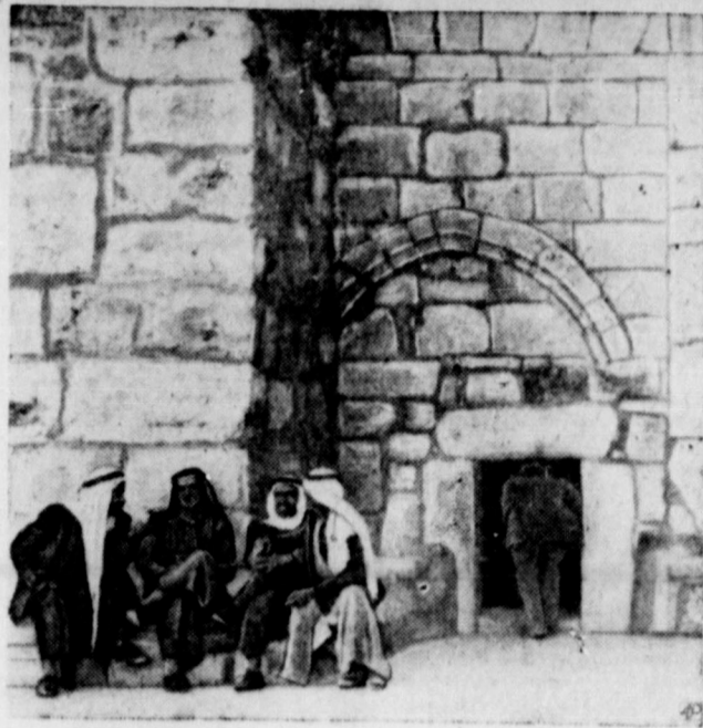
CHRISTMAS SHRINE — Entrance of The Church of the Nativity in Bethlehem where Moslems and Christians both pray. The pattern of the stones shows how the door was once much larger, but was reduced to keep out livestock.
