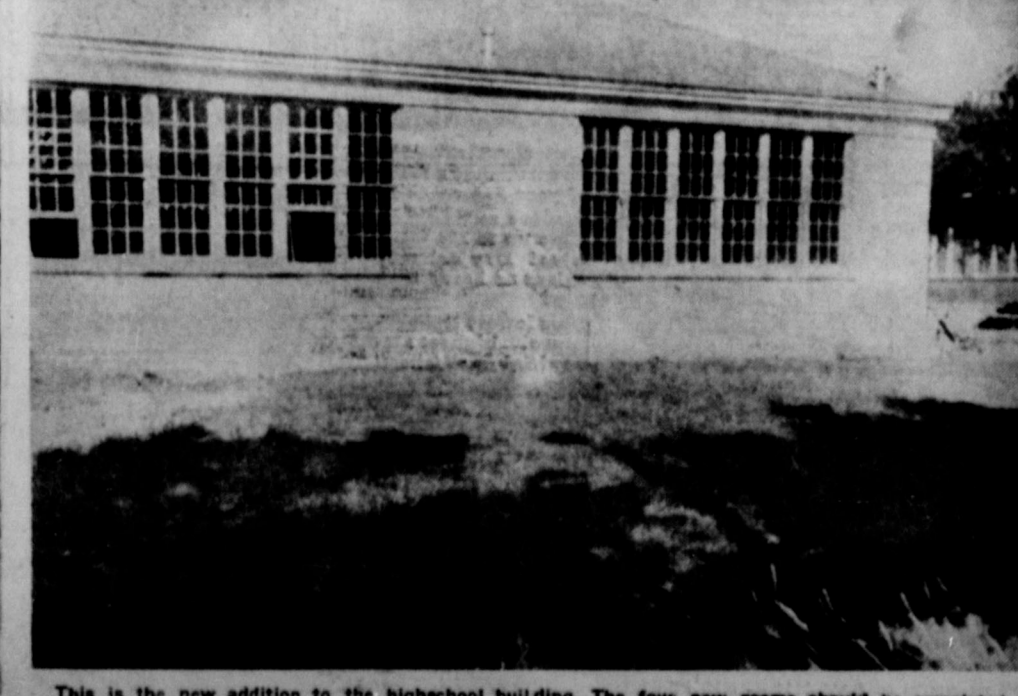
This is the new addition to the highschool building. The four new rooms should be completed by next week.
