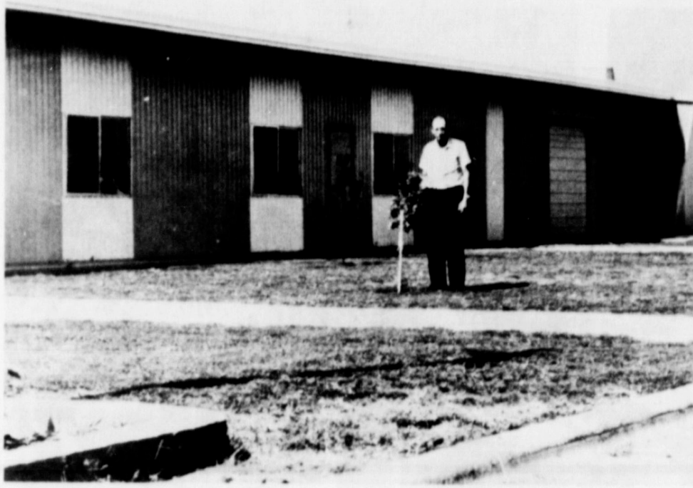
LANDSCAPING OF THE SHOP GROUNDS was recently completed, and the grass has been fertilized and watered, adding beauty to the school campus. Supt. Bill Mann is shown looking over the recent improvements.
