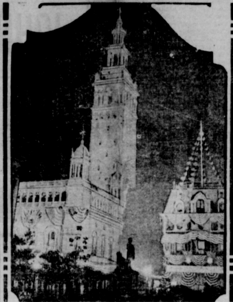
View of the Madison Square garden at night showing the illuminations. The lighting scheme was arranged by the engineers of the Westinghouse Lamp company, co-operating with the New York Edison company, and is a part of the city's welcome to the visiting delegates.
