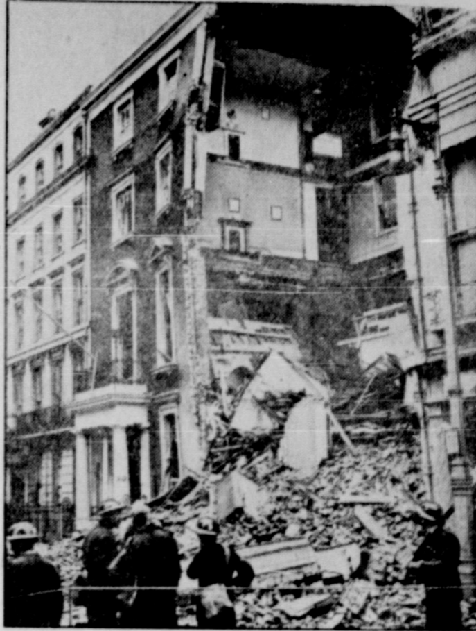
Force of explosion of Nazi bomb was enough to break the wall out of this four-story London apartment building, but didn't shake the pictures off the walls. Men in helmets are A. R. P. workers.
