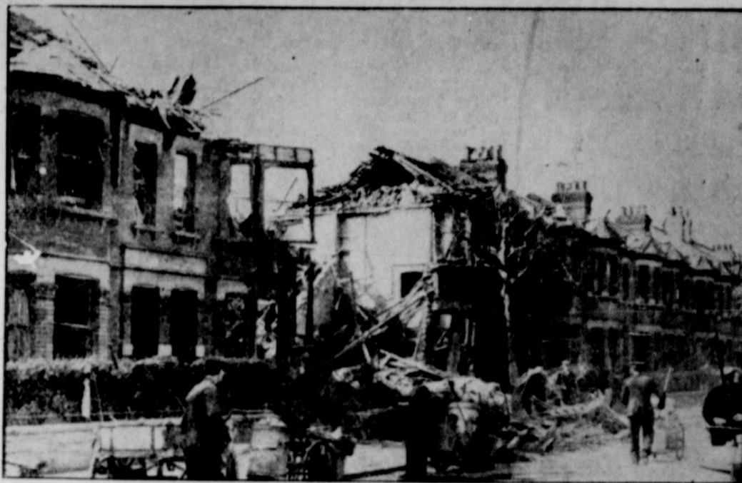
Repair squads tidy up streets in London area after fierce raid by German bombers. Note roofs blown off several houses by explosion of bomb which fell in the center of row.
