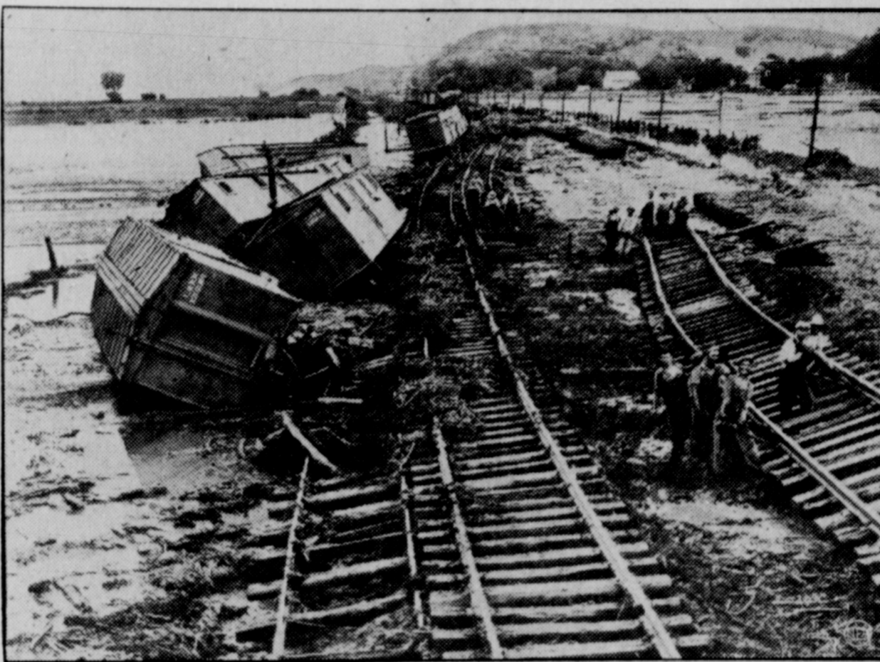
Prayers of Iowa farmers for rain were answered a hundredfold when the heavens gushed and damaging floods swept the state, parched by months of drought. Here is a remarkable picture of the toll taken by the deluge, the wreck of a train caused by washout of tracks near Council Bluffs, Ia., when Honey creek became a raging torrent overnight. With cars spilled from the rails and flood debris littering the tracks, workmen are toiling to reopen the way for trains.
