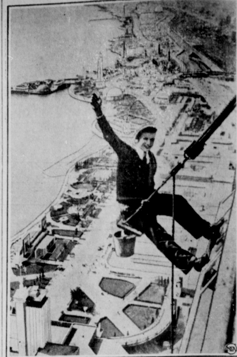
Joe Hrab will probably see more of Chicago's Century of Progress this year than anyone else, for his job is washing windows on the Sky Ride tower. Here's Joe with 600 feet of very thin air between him and the fair grounds, spread along the Chicago lakefront below.
