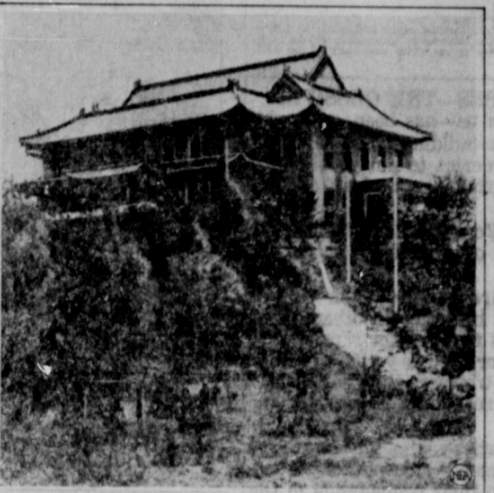
China's $100,000 "White House" at Nanking will be ready for occupancy before Christmas, after two years' construction work—but the occupant is uncertain. It may be Lin Sen, China's president, or it may be Gen. Chiang Kai-shek, actual government head. The mansion, shown here, is built in purely Chinese style, with yellow brick walls and blue glazed tile roof.
