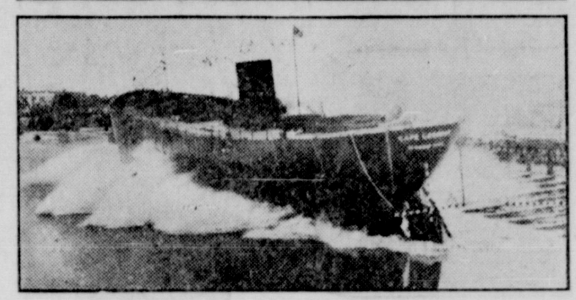
When the U. S. maritime commission's new $1,900,000 cargo ship, Cape Lookout, splashed into the waters of the Neches river at Beaumont, Tex., the ways were well greased with two and a half tons of over-ripe bananas. The bananas, shown being cut by workers in top photo, provided a cheaper lubricant than ordinary grease. This was first freighter launching with bananas, though many smaller ships have used the banana method.
