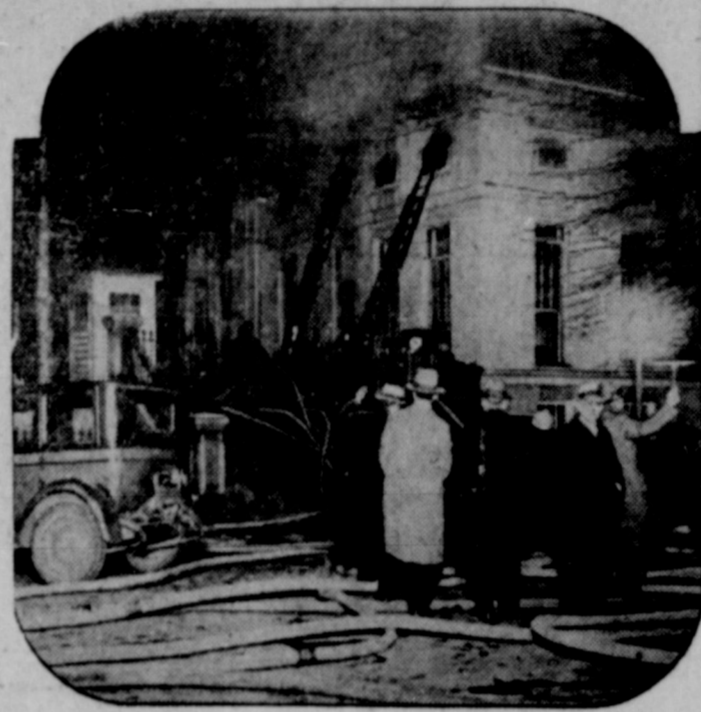
President Hoover's executive offices were ruined in a White House fire Christmas Eve which brought damage to the extent of $60,000. Immediately afterward, the president ordered reconstruction started. Meanwhile, the nation's executive business is being conducted in the living quarters of the White House.
