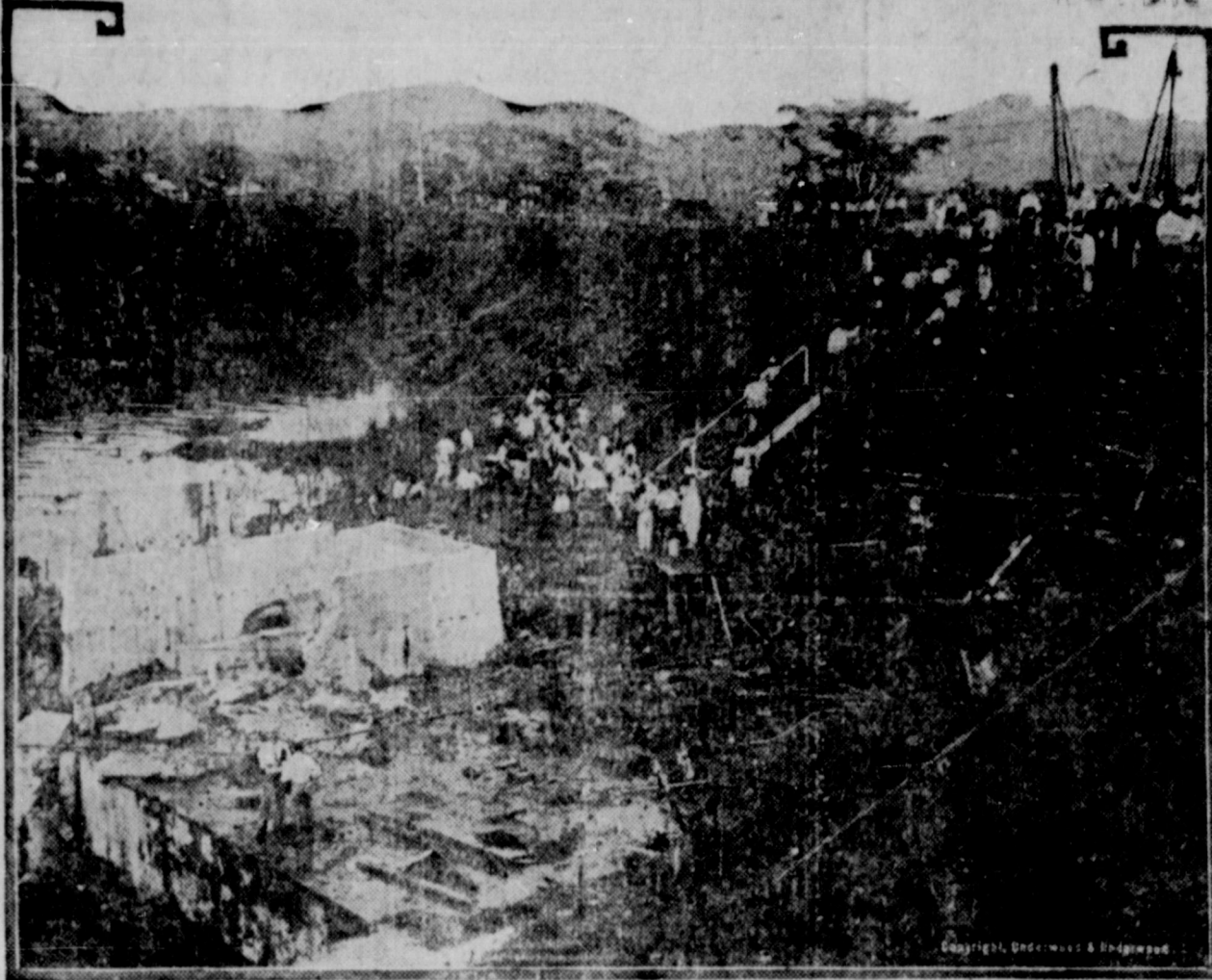
Before the blowing up of the Gamboa Dike a certain amount of water was let into the Culebra Cut through pipes in the dike, in order to form a cushion for the great explosion.
