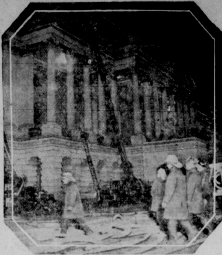
Just ten days after a blaze which almost wrecked the White House executive offices in Washington, a fire broke out in a room near the rotunda of the capitol building, shown above. Charles Moberly, one of the artists decorating the capitol, was found in the room overcome by smoke, but was revived. Repair work is now under way.
