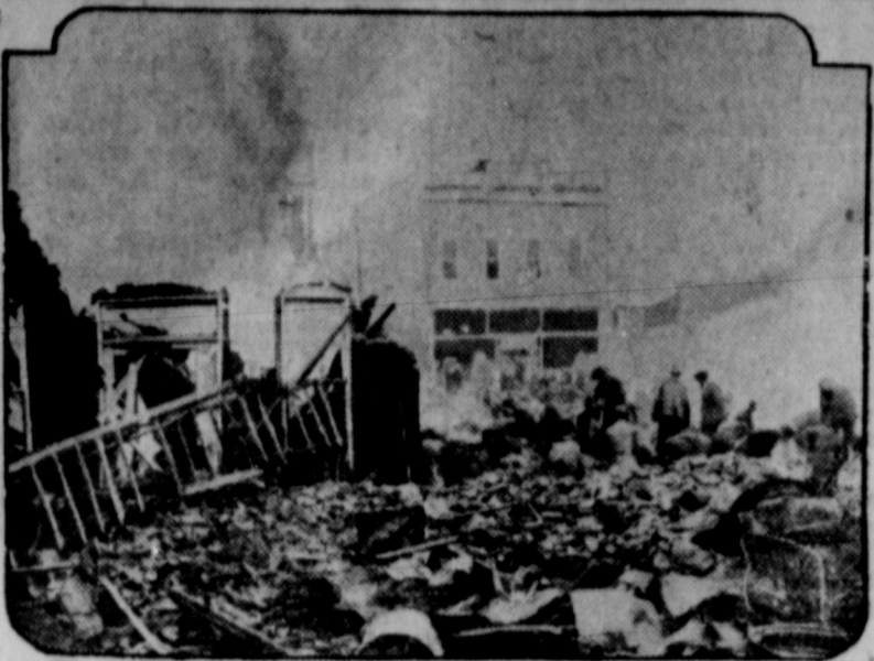
When the mysterious blast reduced a dance hall at West Plains, Mo., recently to this pile of debris, it killed 41 and injured 20 persons. The picture shows volunteer workers searching among the smoking ruins for bodies of the victims. Police are working on a plot theory.
