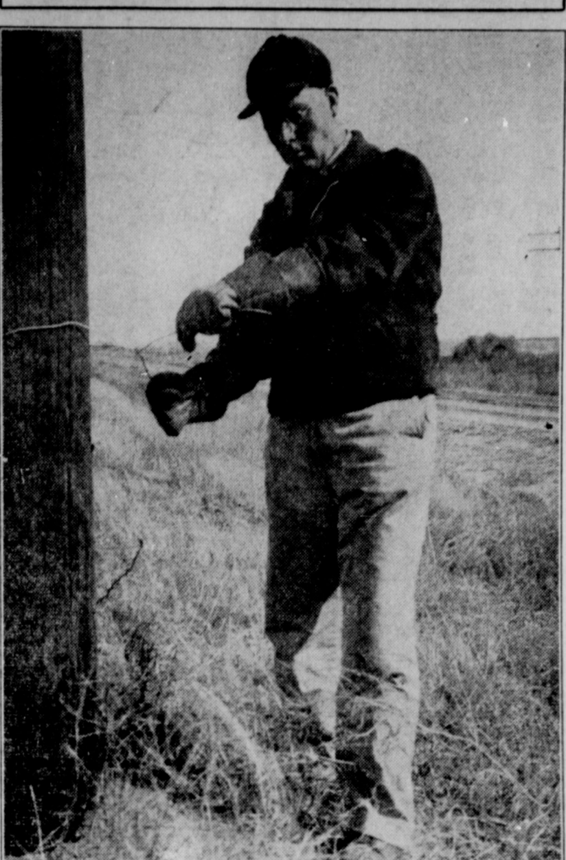
Lineman J. B. Handley of Childress shows how ordinary fesse wire was used for climbing hooks in emergency that won national honors.
