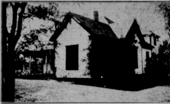
Pictured above is the Odom Sanitarium which will open about the tenth of the month. It is located on South Eighth street at the end of the pavement. Coincident with the opening of the sanitarium on October 10, Dr. J. A. Odom, who will head the institution, will close his offices in the Hall County National Bank building, and will thereafter be found at the sanitarium.
