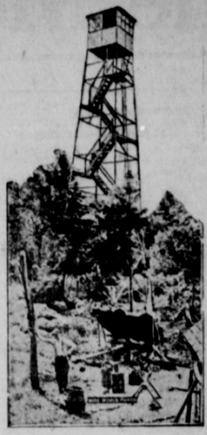
Steel tower in which watchmen are stationed to keep guard over the forests of Minnesota, built to withstand the flames which often destroyed the older wooden structures.
