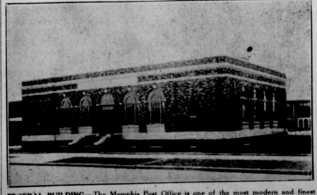
FEDERAL BUILDING —The Memphis Post Office is one of the most modern and finest buildings in the city. The building is conveniently divided into the various departments, where service from each can be more easily rendered. In addition, the postmaster, J. H. Read, has a private office where he may transact business of the post office.
