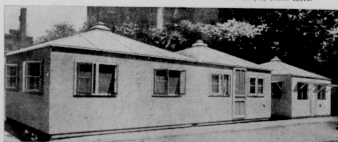
Photo—Washington Star At 11:10 a.m. the workmen had constructed the home, as shown above.
