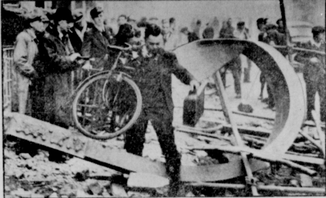
Finning his path blocked by debris in a London street, this bicycle rider carries his vehicle over a twisted girder before proceeding on his way. Damage was caused in a Nazi night raid.
