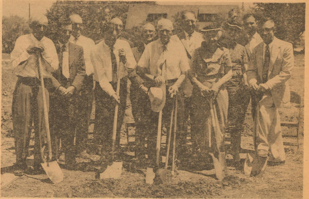
FORMED early in 1958, the First Christian Church congregation held their initial meetings in the Memorial Building. By July of 1959, this ground-breaking ceremony for the new church building was held. Shown left to right are C. L. Martin, Edgar Sauer, L. Kinser, Bennie Harkey, Charles Coombes, Rev. Pearce J. Burns, J. C. Carr, Rev. Thompson, Mrs. J. C. Carr, Mrs. Burns, Joe West, and Bernard Carr. Photo from Success files.
