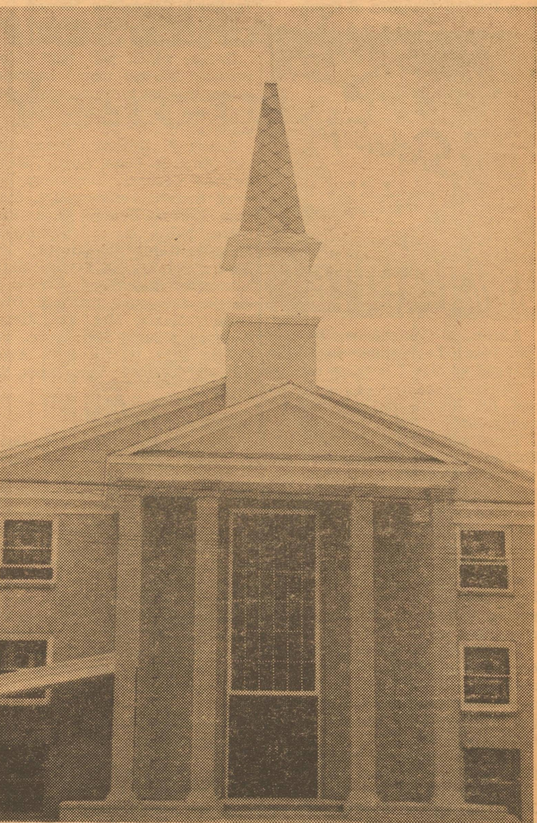
THIS IMPOSING FACADE of the First Baptist church represents a gracious blending of the old building, which was erected in 1928, and the new glassed-in porch with its brick columns and covered walkway at the side that leads to the new annex. —Staff Photo
